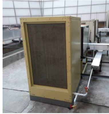
b) Outdoor side heat exchanger
